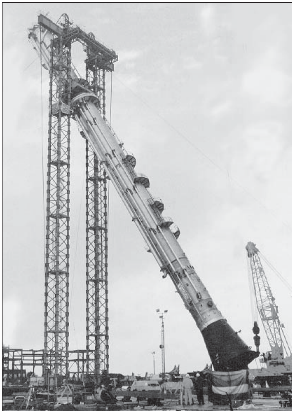
Figure 5.7-2 Gallows Pole Arrangement
