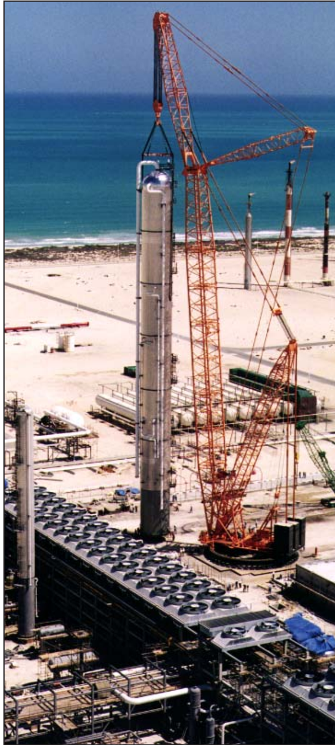
Figure 3.6-2 Ringer Attachment
